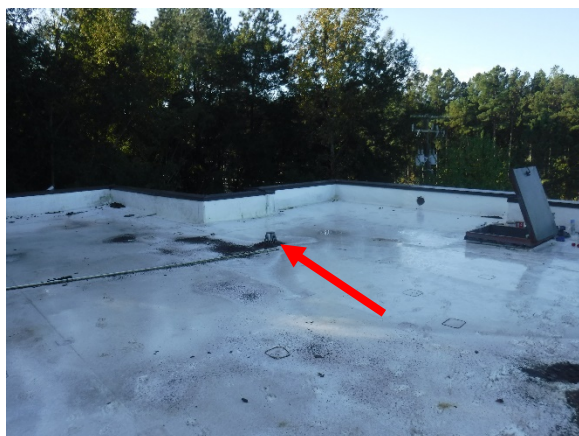
Photo 1. Lead Shielding Under Roofing Membrane at Roof Drains
